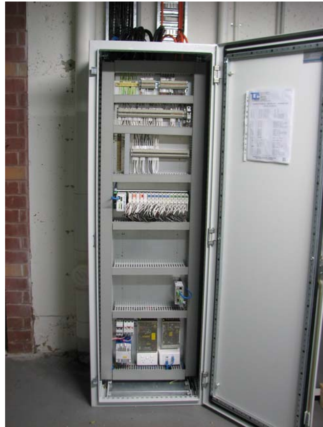
PID-maintained positive air pressure keeps airborne germs out of the operating room.
