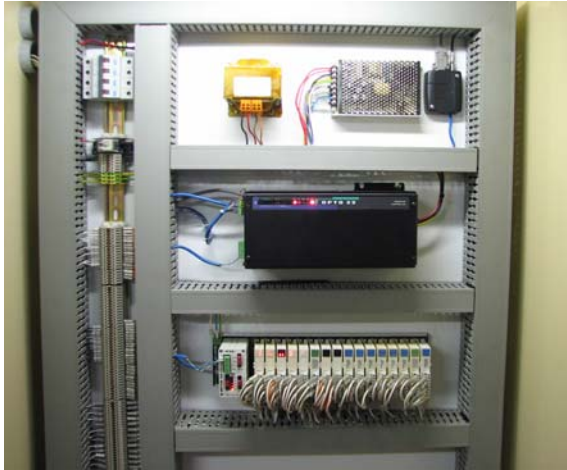
M4s are replaced with SNAP PACs without having to touch any remote I/O or sensors.
